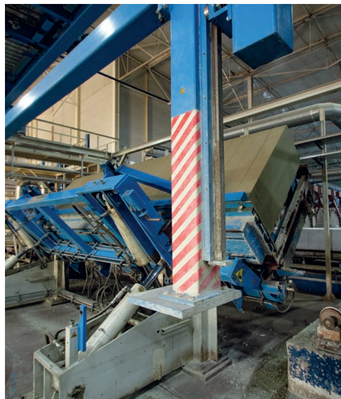
The tilting system rotates the upright cake into a horizontal position before it is stacked with other cakes to start the autoclaving process
