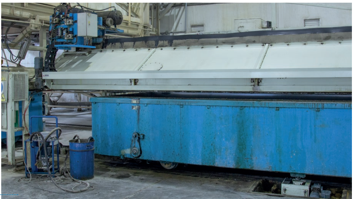
Moulds travelling under the grey Münstermann system to be automatically oiled with a form release agent
